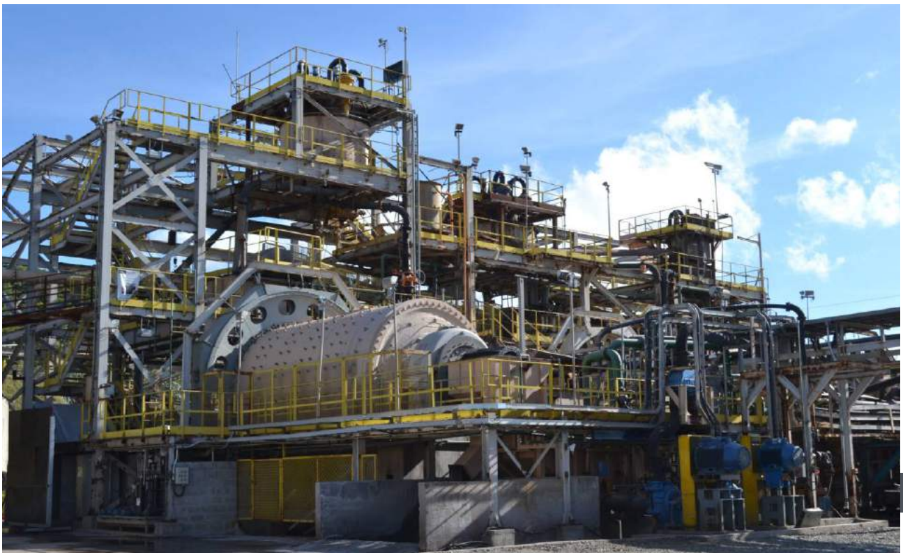
Processing Plant - MTL / Jaguar Mining File
