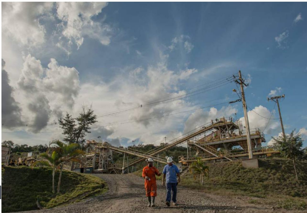
Processing Plant – MTL Unit / Jaguar Mining File
